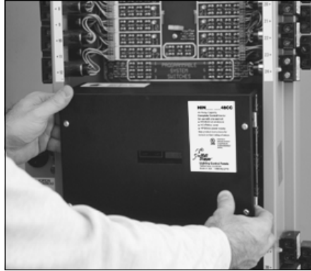
Remove the card cover if installing in a Complete Control interior in order to access the power supply mounting opening.
