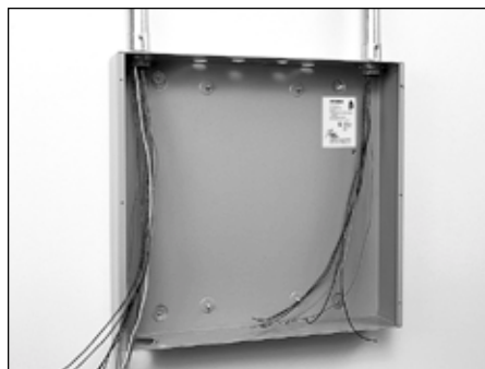
Route wiring through the top, bottom or sides.
