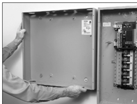
The tub should be level, plumb and rigidly mounted.
